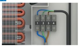
Connect the mains cable from the LED Driver (Input) into to the AC unit live feed so that power is suppled when the AC unit is on, this should be done by a qualified electrician.
