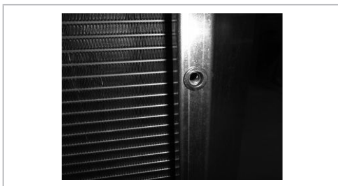
Fig. 2: Points de suspension de charge M8x30 (max.)
